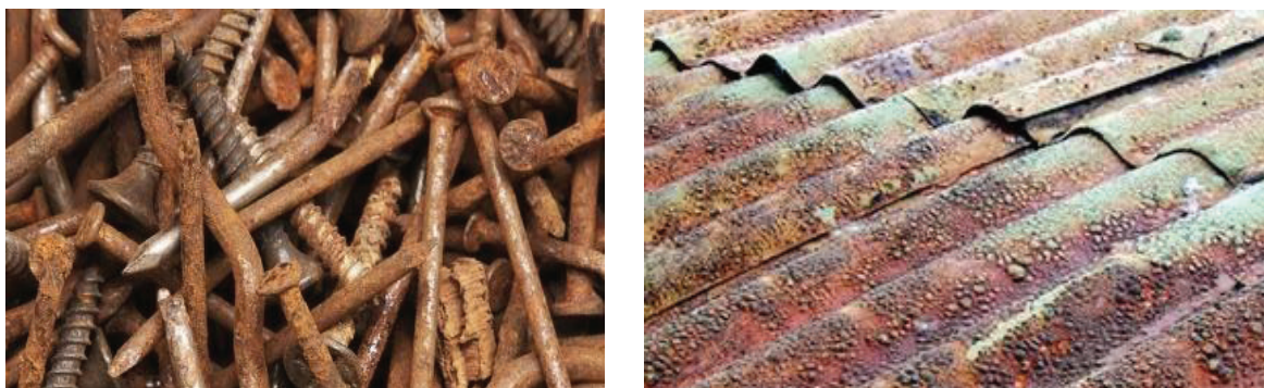
Figure 10.10: Rusted nails and iron sheets
