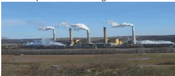
Oil-fired power station in Uganda
